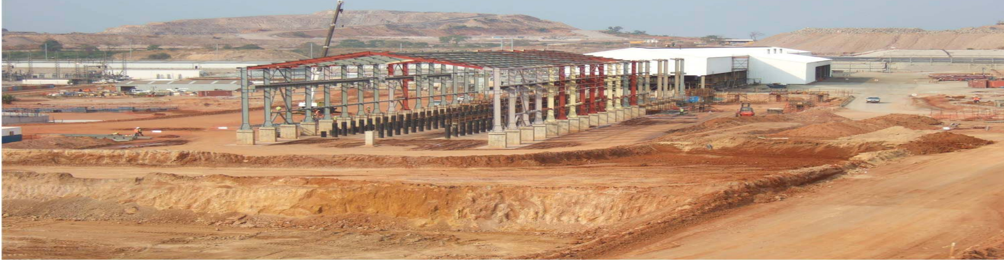
SX Retaining Wall
