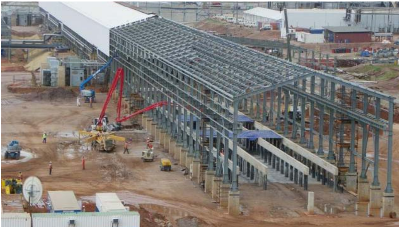
Tank House Expansion
