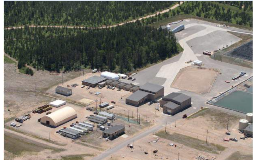
Mine site facilities
