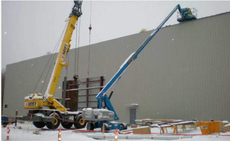
Mill site facilities
