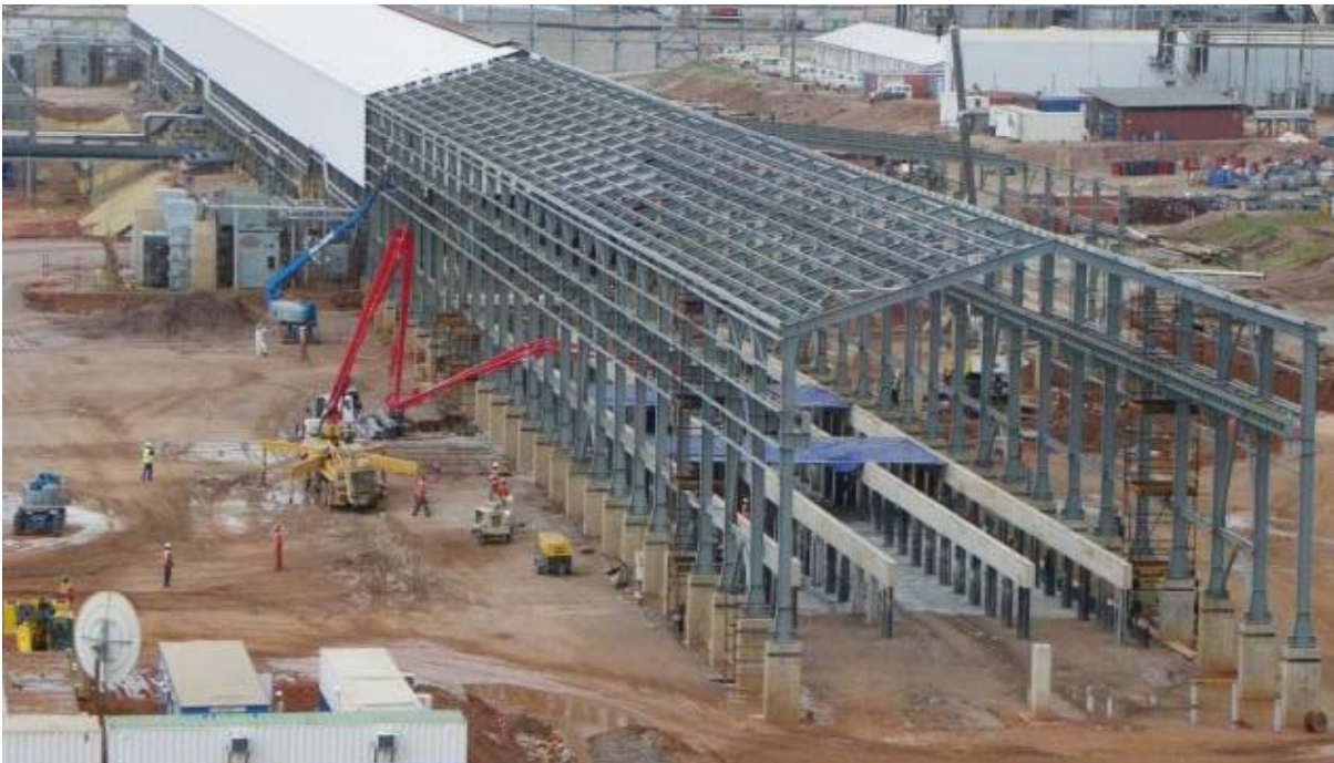
Tank House Expansion
