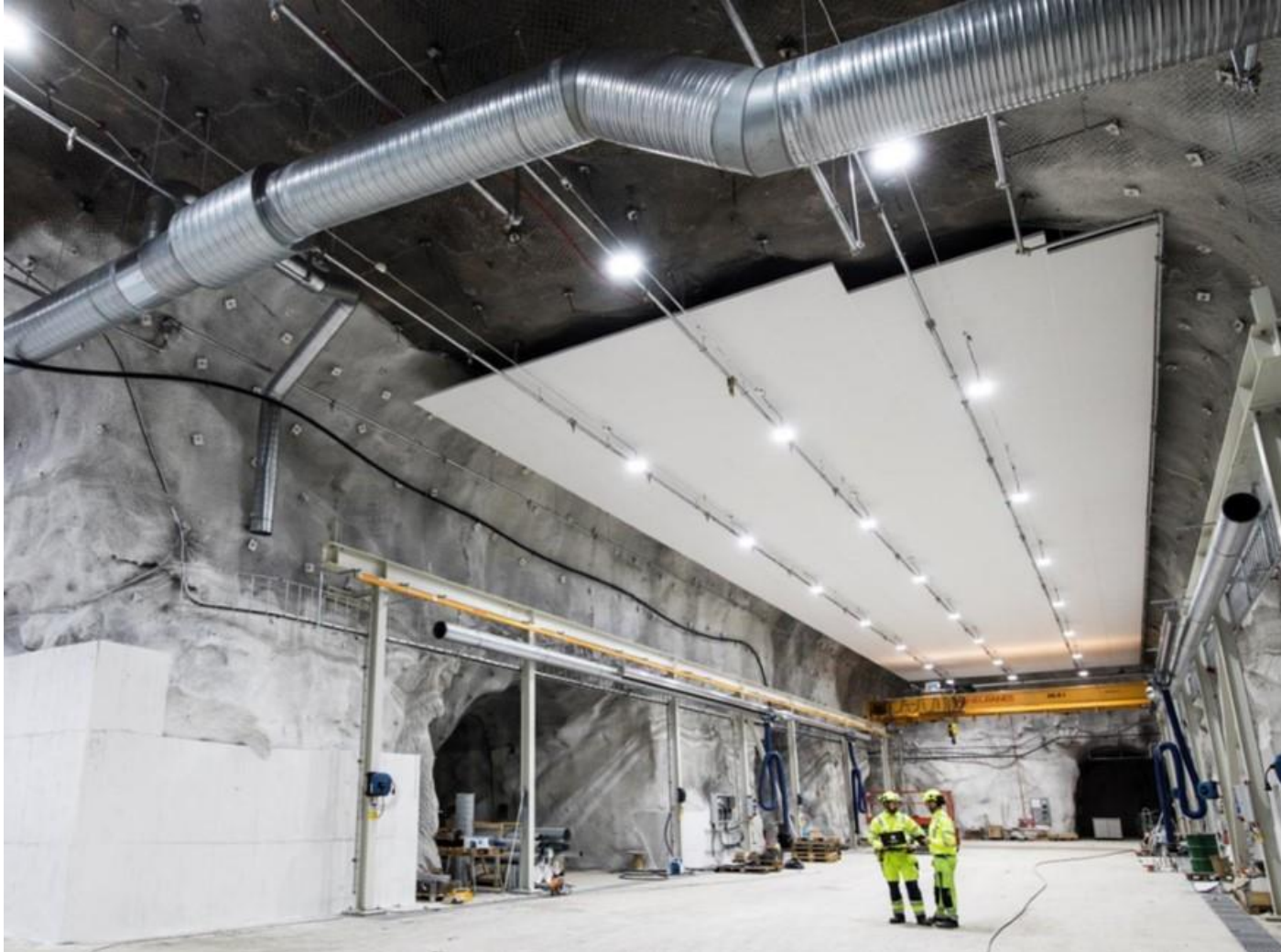
Construction of new 1140 level service area in Zinkgruvan mine
