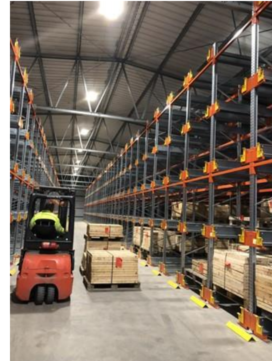
New Zinkgruvan core shed completed in Q4/19
