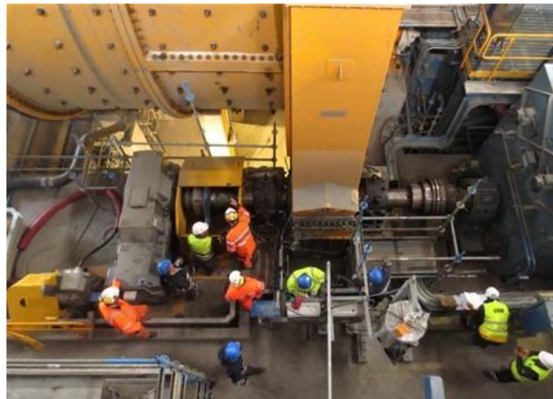
SAG mill commissioning work
